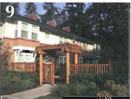
9 Multi-family building, 2-story
