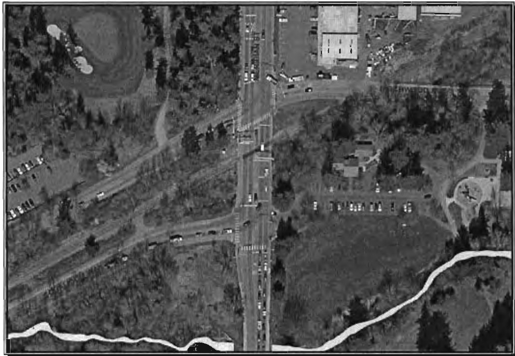
Figure 1 above shows the existing intersection geometry and traffic signals
