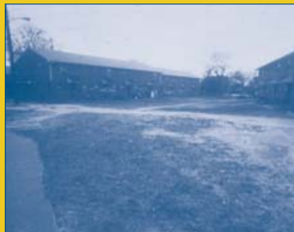
Diggs Town – before
