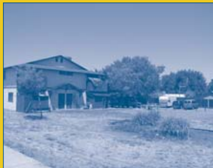
Poorly maintained property
